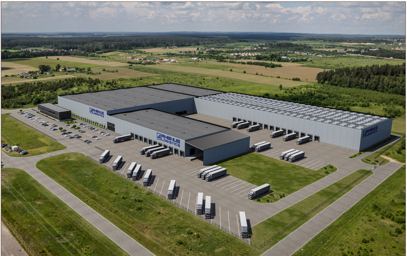
BSP Park - Vilnius A4 (top) | Photo of current terminal. BSP Park - Vilnius A4 (bottom) | Illustration of terminal after planned expansion.
