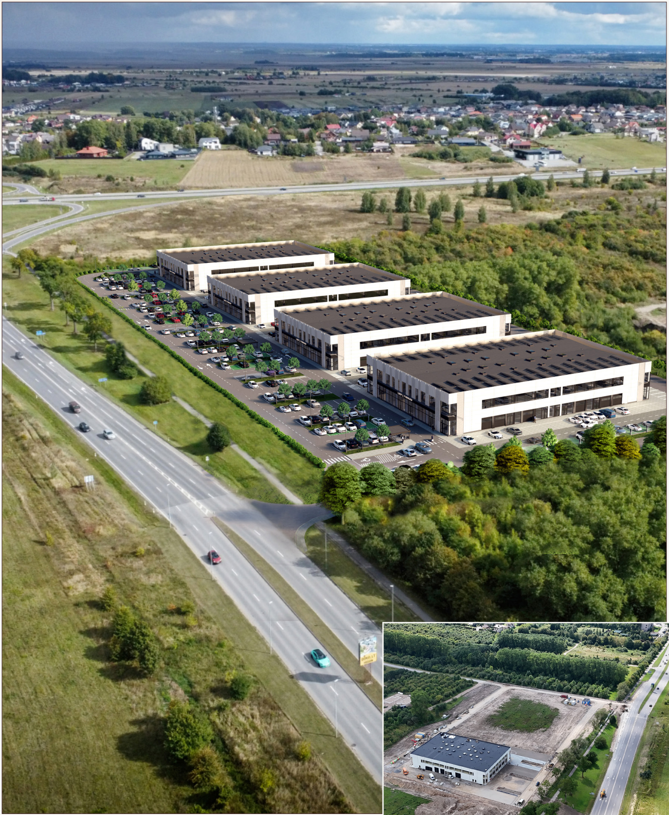
Large frame | Concept visualisation of Liepų Parkas (retail and business park, Liepų Street, Klaipėda) Small frame | Construction in progress, August 2024
