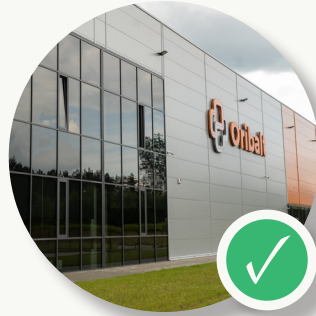
Oribalt terminal BREEAM In-Use: "Very good"
