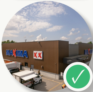
Maxima retail stores BREEAM In-Use: "Good"
