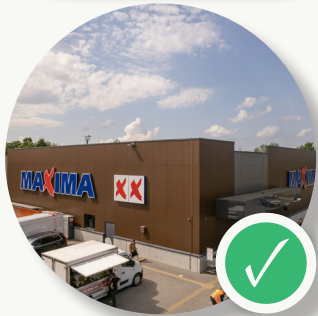
Maxima retail stores BREEAM In-Use: "Good"
